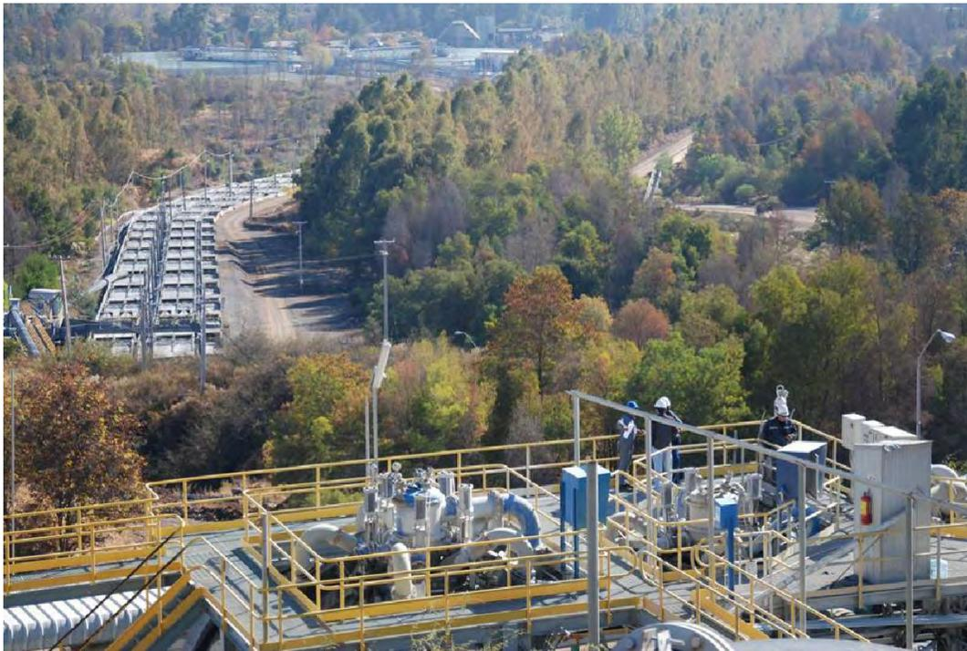
**Photo 4-4: Photograph of the MVC Thickeners, Moly Plant and Offices**
